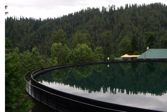
Rain Water Harvesting
